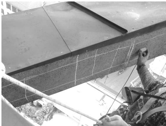
Figure 10 – Detection of the rebars.
