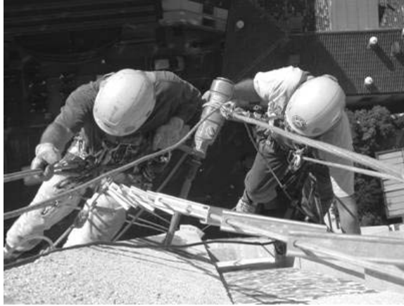
Figure 9 – Inspection team at work.
